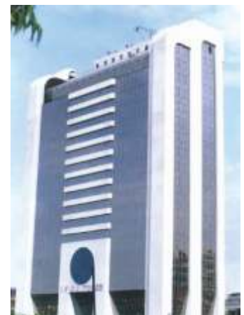
IFCI BUILDING 26 FLOORS OF STEEL STRUCTURE COMPLETED IN SIX MONTHS
