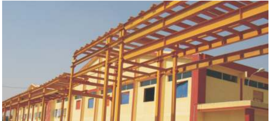
HEAVY DUTY CABLE STRUCTURE FOR HOTLINE
