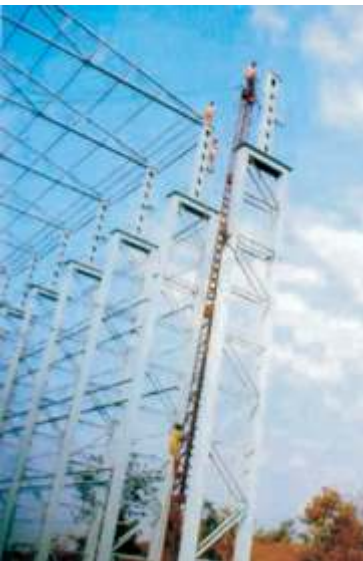
HEAVY DUTY CRANE STRUCTURE
