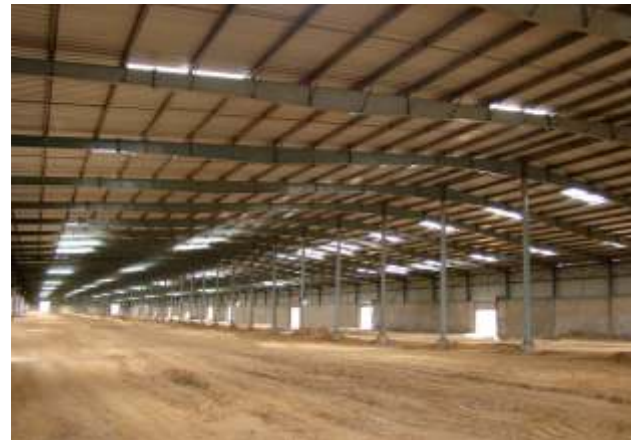
INSIDE VIEW OF 350 MTR. LONG PEB FOR M/S ROYALE LOGISTICS, NEAR GURGAON
