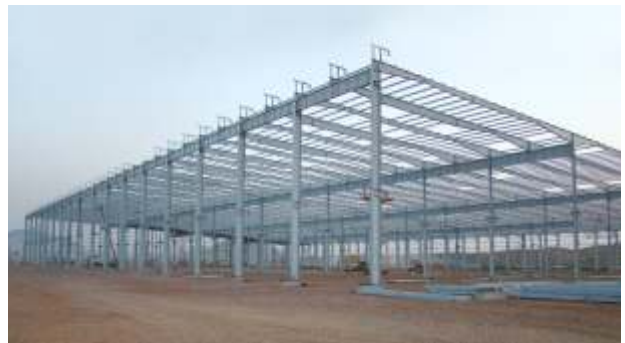
THE PEB WAREHOUSE IS 280MTR LONG AND 212 MTR WIDE
