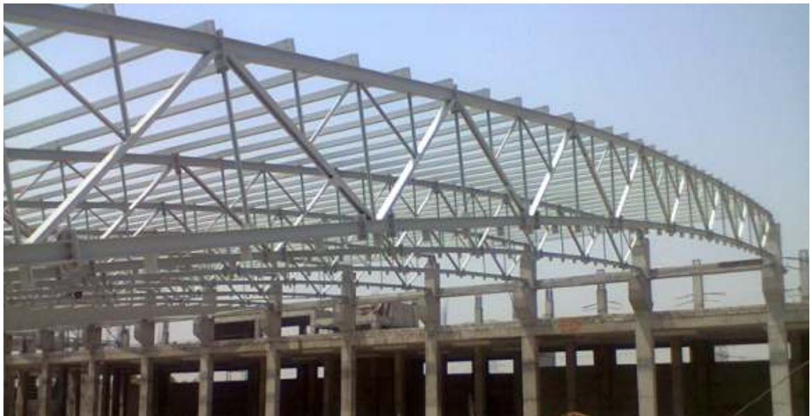
50 MTR CLEAR SPAN CURVED TRUSS FOR KAYEM FOODS AT SONEPAT
