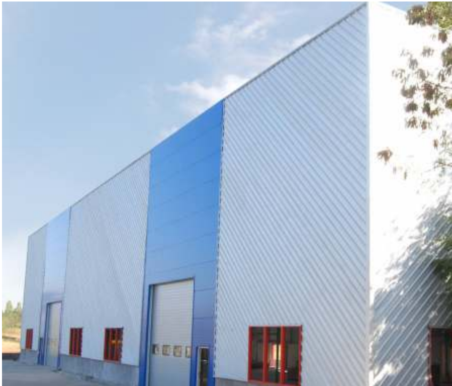
AUTOMOTIVE COMPONENT PLANT, PUNE WITH DIAGONAL PROFILE SIDE & GABLE CLADDING
