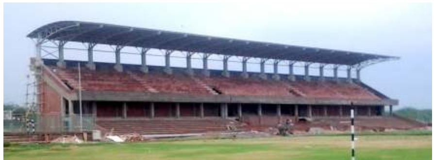
STADIUM ROOF STRUCTURE AT AGRA
