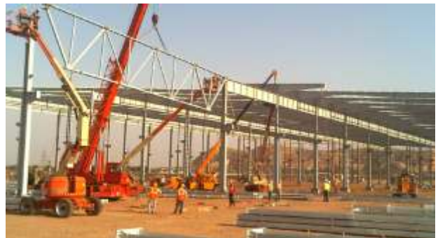
24 MTR JACK BEAM DURING INSTALLATION AT SAINT GOBAIN GLASS INDIA, BHIWADI
