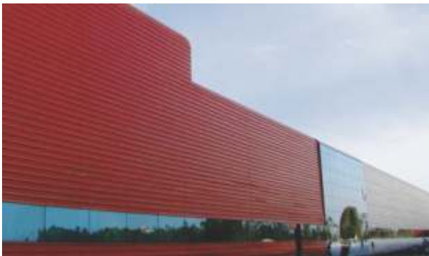
HORIZONTAL/CURVED SIDE CLADDING FOR FLEXITUFF INTERNATIONAL, KASHIPUR
