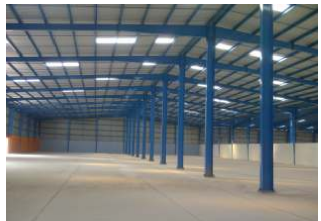
20,000 SQ. MT. WAREHOUSE BUILDING AT GURGAON
