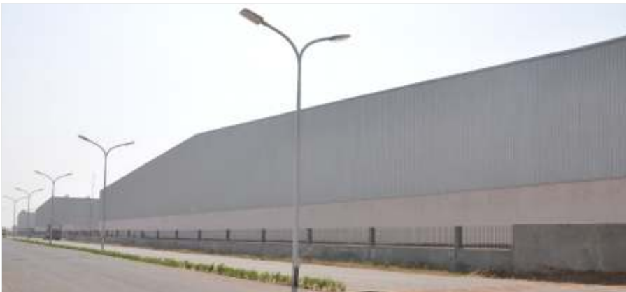
1MILLION SQ. FT. LOGISTIC PARK AT MANESAR, GURGAON
