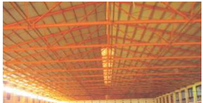
CLEAR 52 MTRS.(171') SPAN STRUCTURE FOR HOTLINE
